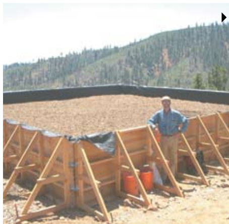
Jim Gusek, Golder Denver, standing next to the pilot scale sulfate reducing bioreactor
