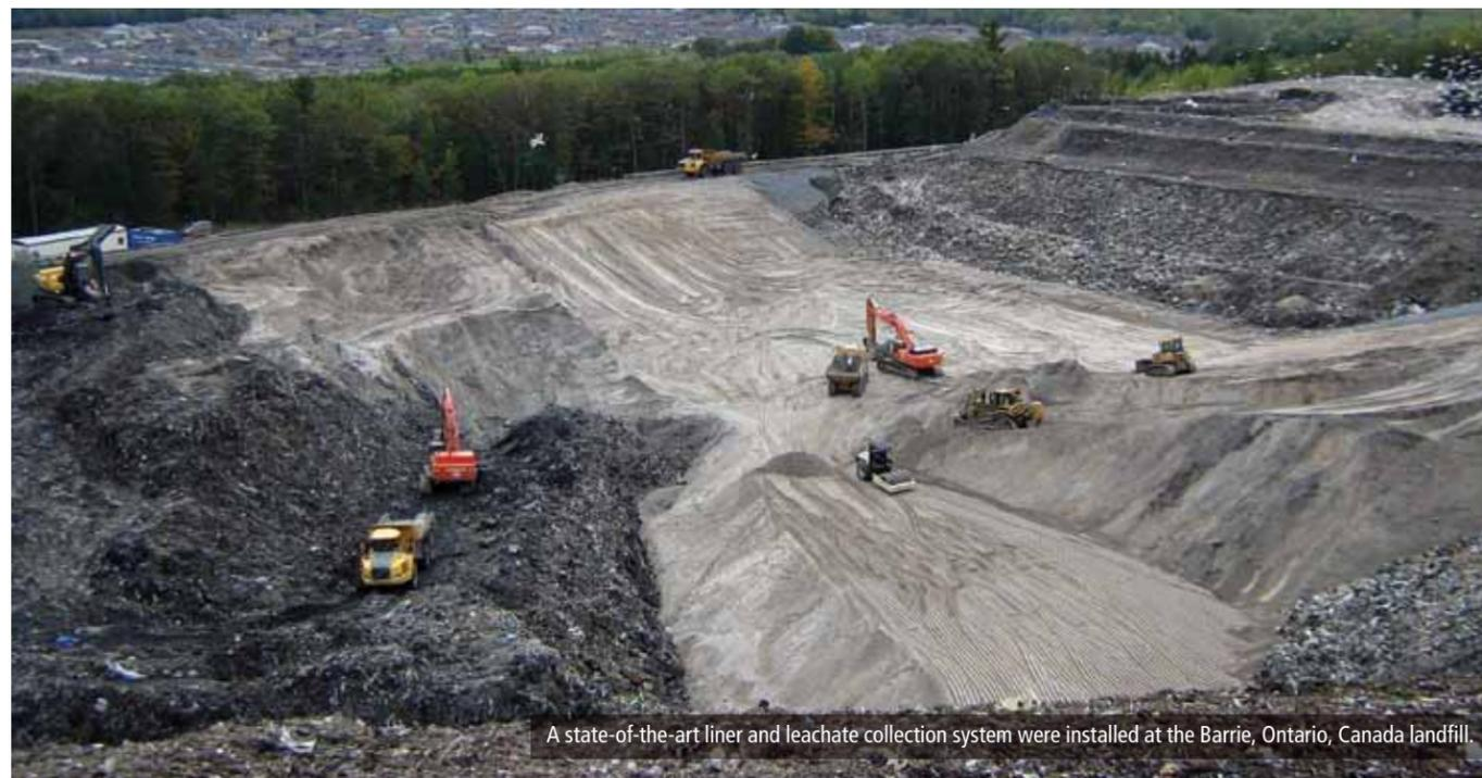
A state-of-the-art liner and leachate collection system were installed at the Barrie, Ontario, Canada landfill.
