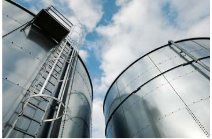
Leachate treatment tanks
