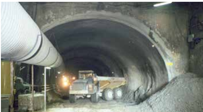
M5 East Motorway, Sydney, NSW
