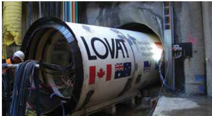
Melbourne Main Sewer Replacement, Melbourne, VIC
